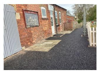
The station platform has undergone some refurbishment: new tarmac surface, picket fence and hard standing for table and chairs.
